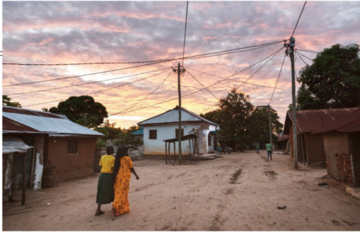
Active and inactive power lines in Matipwili on Jan. 22.
